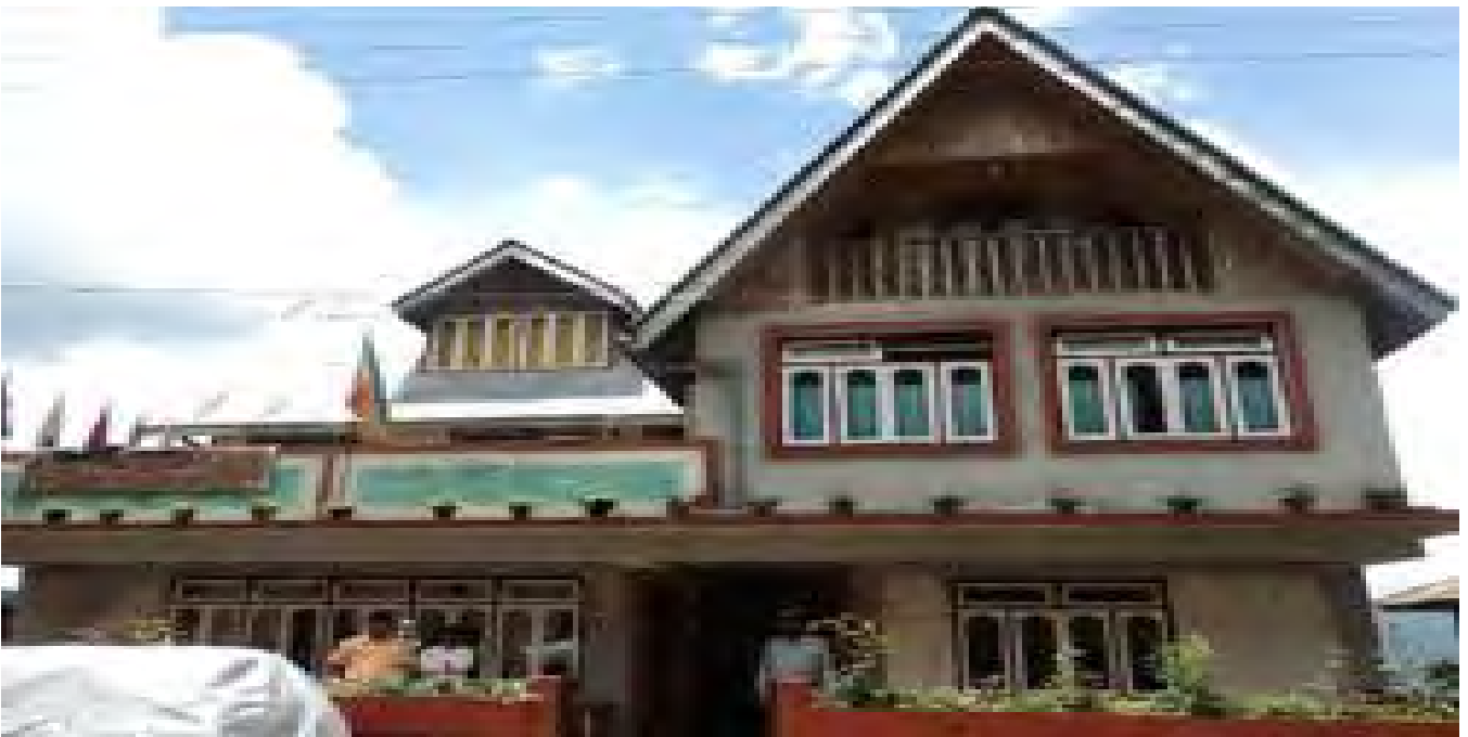
Sada Mangder Site Office
