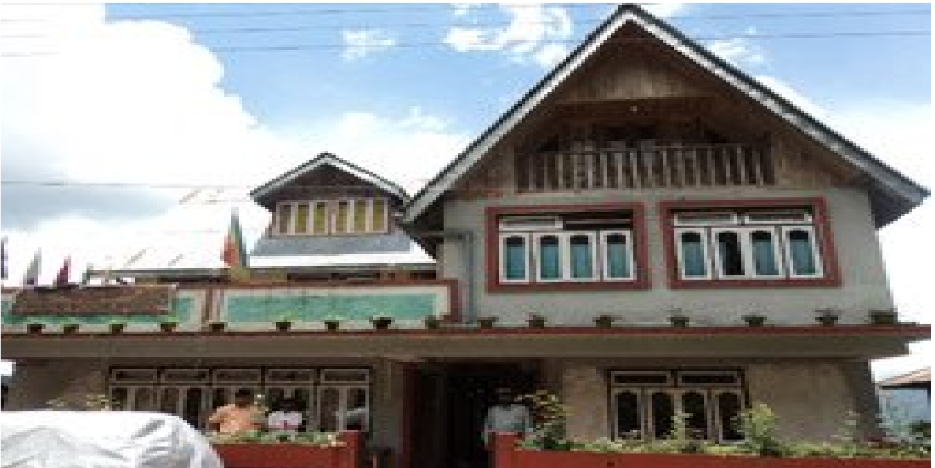
Sada Mangder Site Office
